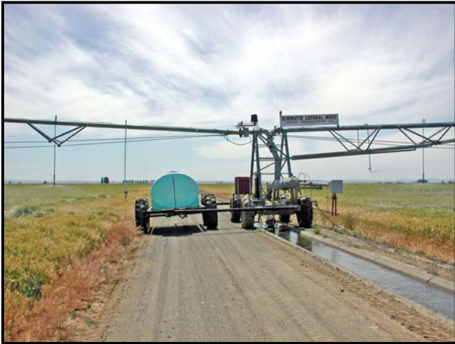
Figure 2. Linear (or lateral) move irrigation system.
